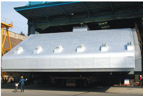
Upper block Insulation
